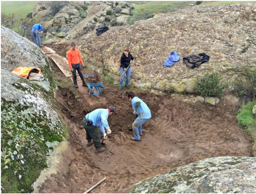
Figure 2. Continued hand removal of soils for a large vernal bedrock vernal pool (#NP-10), Contra Costa County, CA, December 2015. Image credit Jeff Alvarez.
