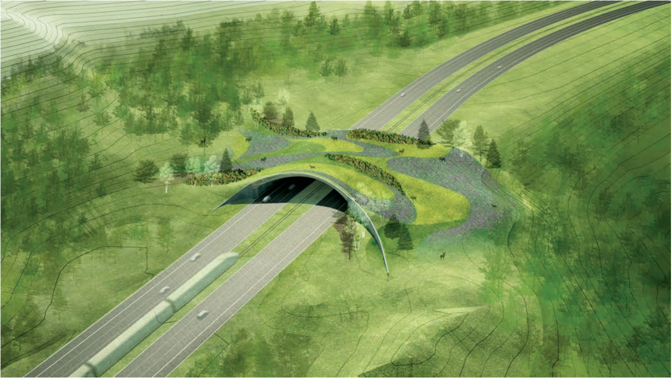
Figure 1. Aerial view of the wildlife crossing and its integration into the landscape. Our proposal extends plant communities found onsite onto the bridge and modifies their maintenance in light of the more severe bridge climate: water availability, temperature, winds, shallow soil, harsh winter climate and proximity to highway. Species have been selected for their tolerance to conditions on the bridge as well as resistance to beetles and other pests. Engelmann spruce ( Picea engelmannii ) and subalpine fir ( Abies lasiocarpa ), with the lodgepole pine ( Pinus contorta ) forests, dominate in this zone. The fairly homogeneous expanses of Engelmann spruce and subalpine forest are interrupted by stands of aspen, grasslands, meadows, or wetlands. Rich diversity and a dense cover of herbaceous and shrub species can be found in the understory of moist groves, while drier sites provide a grassy understory of thurber fescue ( Festuca thurberi ), slender wheatgrass ( Elymus trachycaulus ), and blue wild rye ( Elymus glaucus ). Our structural approach allows the surface of the bridge to undulate with the surrounding landscape and provide areas of deeper soil for trees.
