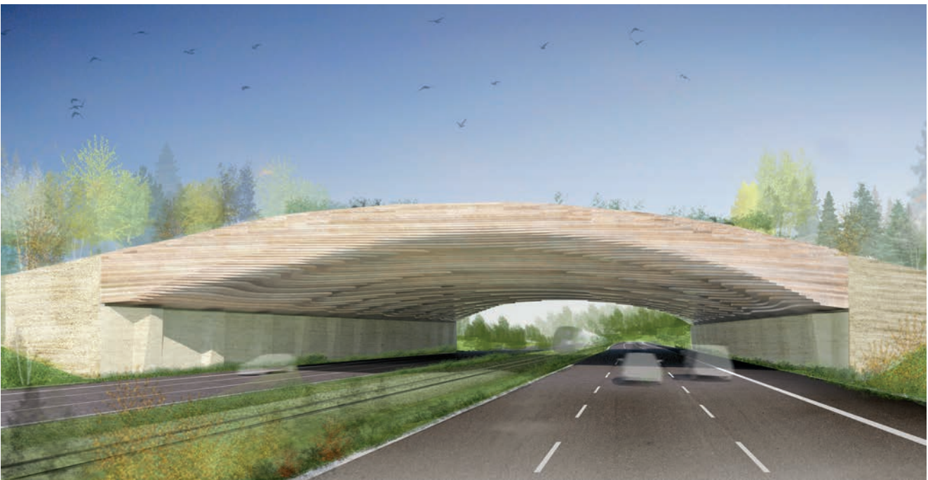
Figure 2. The monolithic bridge corpus is designed as a wide continuous beam. The structural system of the continuous beam is designed with a high redundancy and robustness without any joints.
